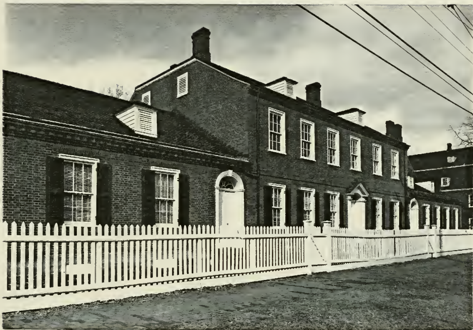
Old Economy Village - Great House, front facade
